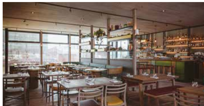
PRECISION LUMINAIRES MOUNTED ONTO RUBBED BRONZE BASIS TRACK RECESSED INTO NARROW TROUGHS IN THE WOODEN CEILING
